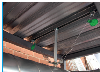
Transverse bracing
