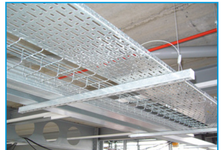
Multiple cable trays on single channel
