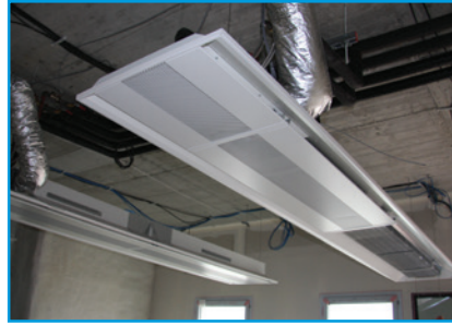
Chilled beams
