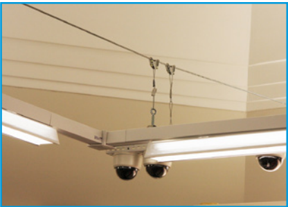
Lighting and Camera on Catenary
