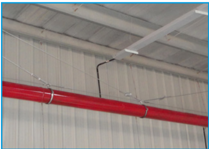
Bracing for steel pipes
