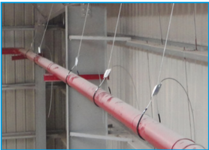
Intermediary supports for steel pipes
