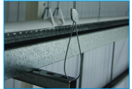
Perforated cable tray on channel
